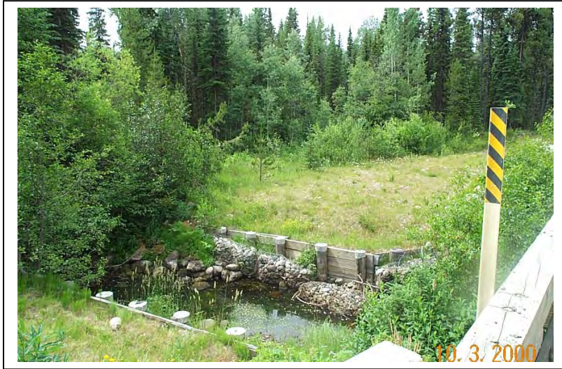
Photograph #1494: De-activated old bridge
