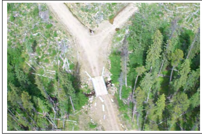
Photograph # 1146: Bridge xing in upper Woodjam
