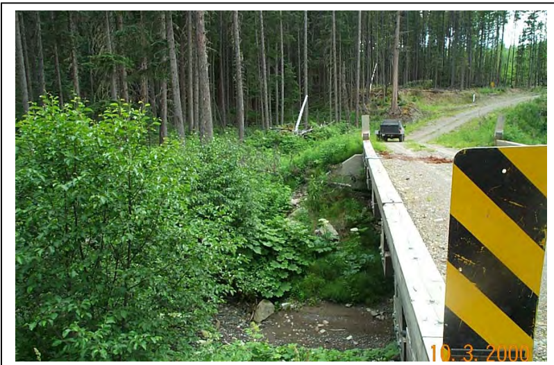
Photograph # 1505: Bridge over Woodjam, SCQI score=0
