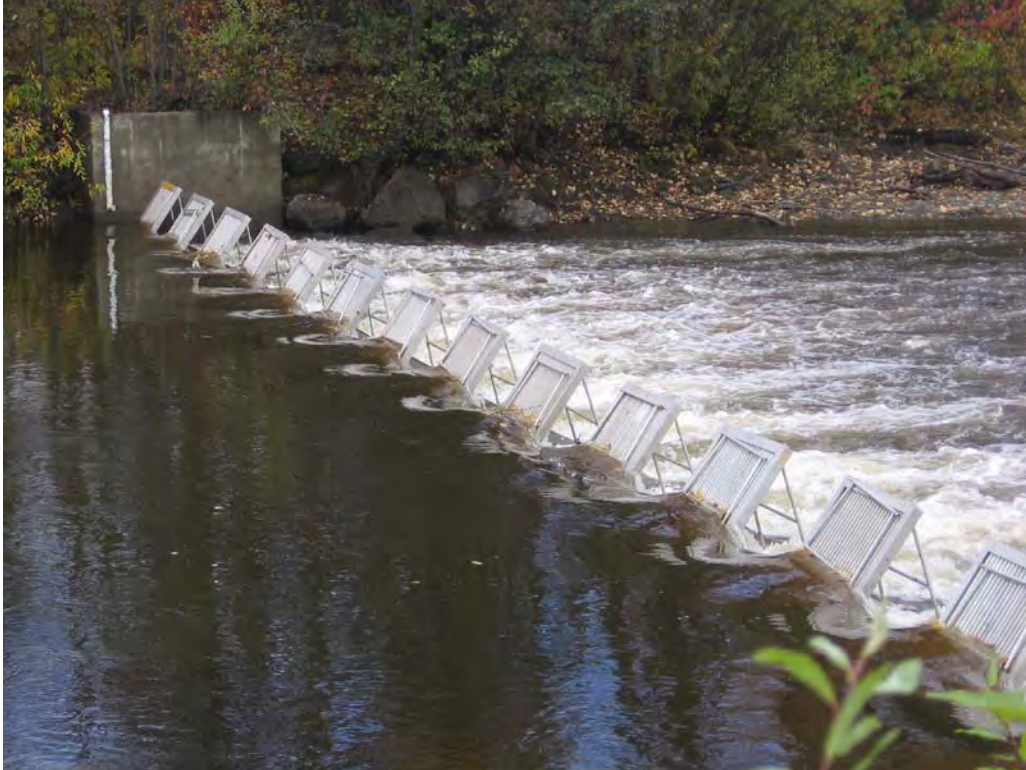
Figure 16: Sockeye diversion fence on the Horsefly River allowing fish passage.
