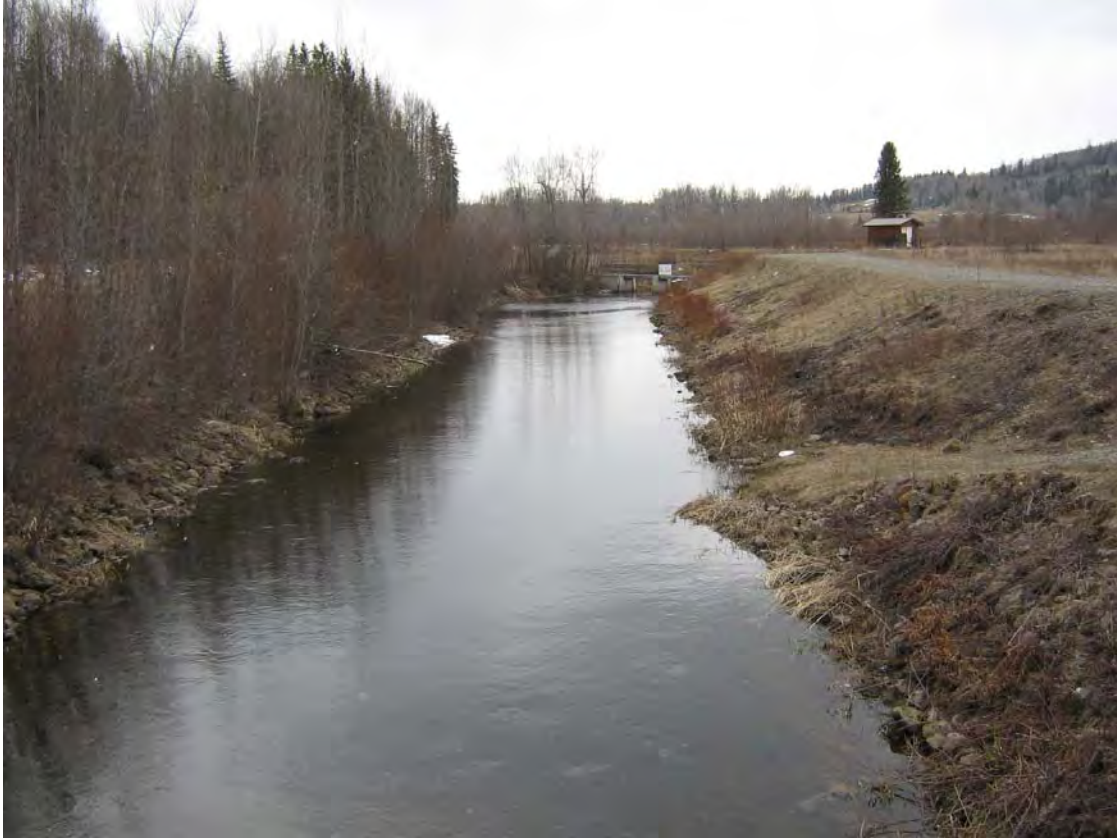
Figure 11: Upstream view of the spawning channel showing the valve house.
